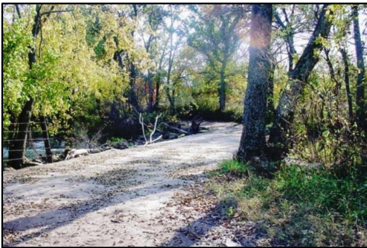
49 Low Water Bridge on Center Creek
